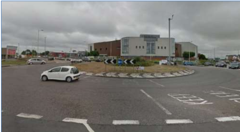
Figure 4 - Westwood Roundabout (A256/A254)
